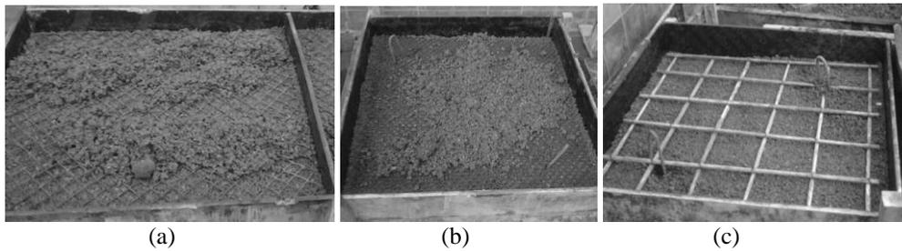
Figure 2. Casting of slabs reinforced with (a) geogrid type I, (b) geogrid type II and (c) GFRP rods
